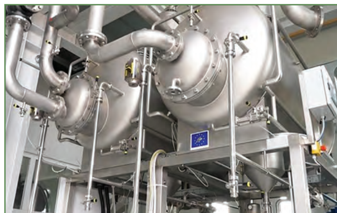
Figure 3b. The Green Biorefinery plant, evaporators, in Japons Austria
