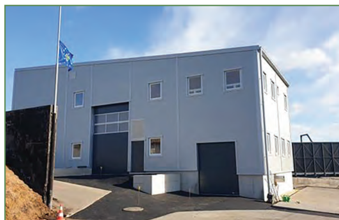
Figure 3a. The Green Biorefinery plant in Japons Austria
